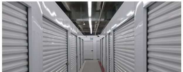
Lockers at the Leaside facility look alike from the outside but colours on the edge of the linoleum floor aid navigation through the maze.
