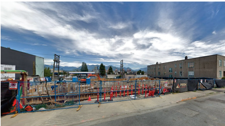
Construction formwork in progress, ground level, July 2018
