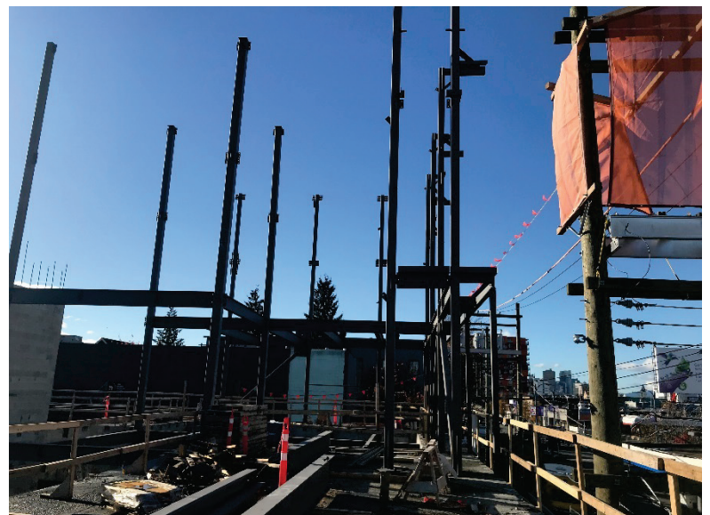
(above) Structural steel install to level 4, November 2018
