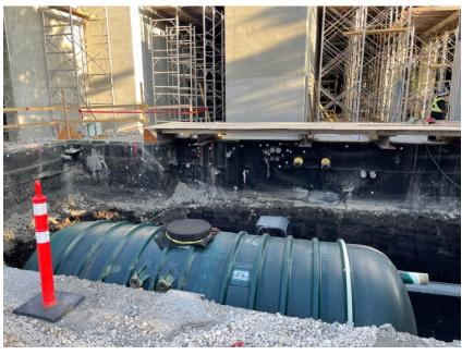
The rainwater reclaim tank has now been installed for car wash. We are proud to say that this car wash will have the first state-of-the-art rainwater harvest tanks in Western Canada. These tanks will be used to collect and store rainwater that will be treated and subsequently used during the car wash process.
